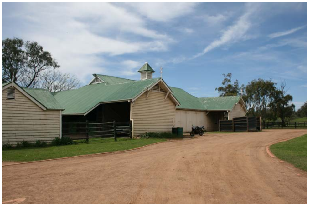
Figure 87 The main stable building, viewed from the north west. The tractor shed is shown in the left foreground source: Heritas 2011
