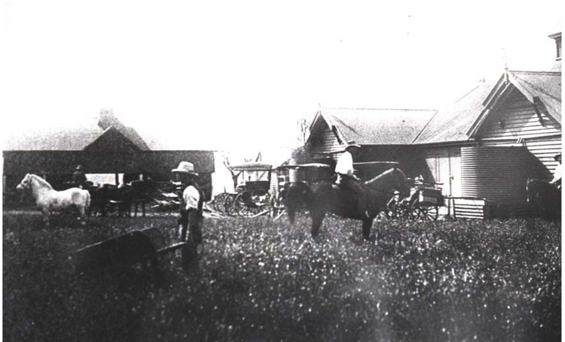
Figure 57 The stables complex, viewed from the south. source: copied from negatives of images held by historian Rosemary Annable
