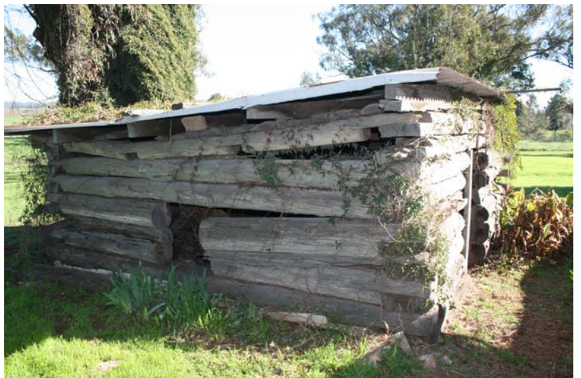
Figure 94 The log structure, viewed from the south east. source: Heritas 2011
