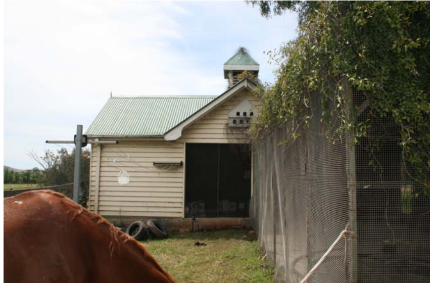
Figure 82 The dovecote, viewed from the south west. source: Heritas 2011
