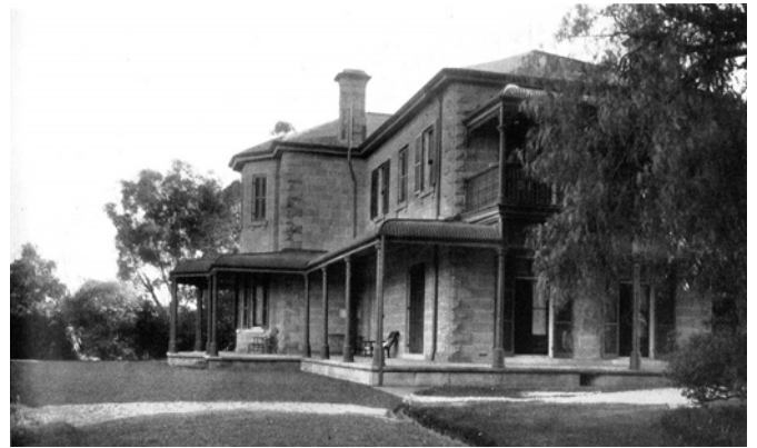
Figure 59 The south western sector of the house, with Pepper tree at right. source: Pastoral Homes of Australia, 1931
