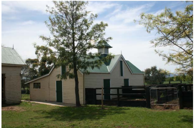
Figure 88 Stable 2, viewed from the south. source: Heritas 2011
