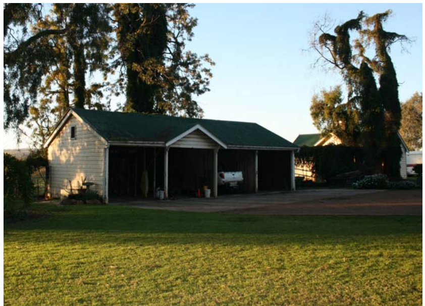
Figure 81 The carport, viewed from the south west. source: Heritas 2011
