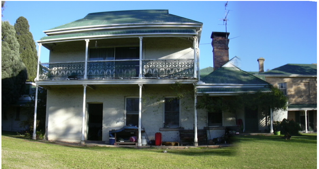
Figure 72 Servant's Quarters, from the north. source: Heritas
