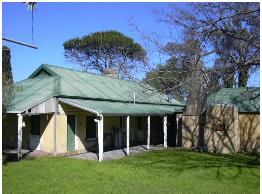
Figure 92 Rous Lench homestead, viewed from the north east. source: Heritas 2011
