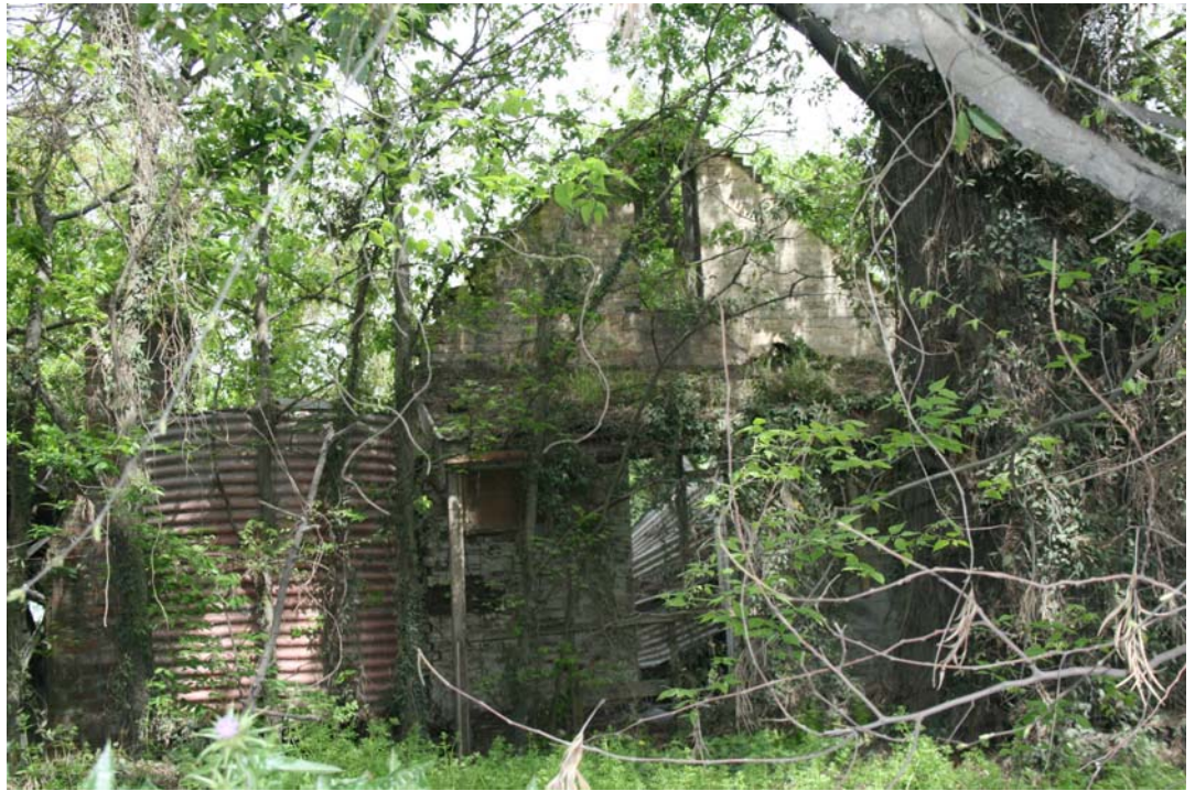
Figure 99 The gardener's cottage, viewed from the east. source: Heritas 2011
