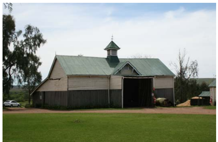
Figure 83 The hayshed, viewed from the south west. source: Heritas 2011
