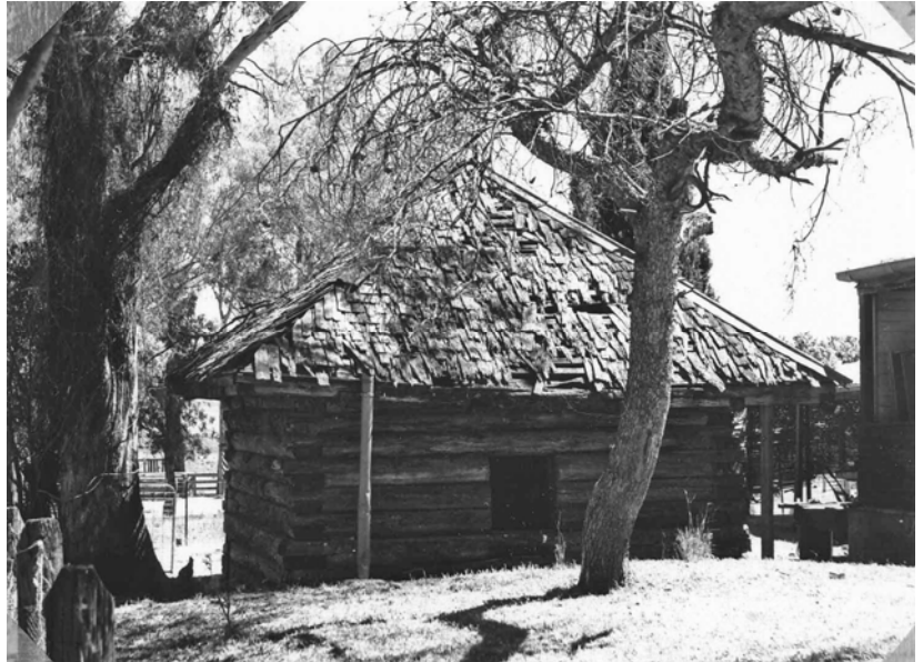
Figure 50 Part of this building constructed from undressed timber remains at Rous Lench but a piece of flat corrugated iron has replaced the shingle roof. Its purpose is unknown. source: National Trust Listing Files
