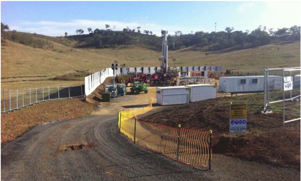
Figure 5.2-40 Typical Access Track and Drill Rig on Hardstand Pad
