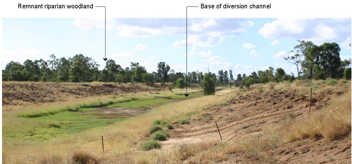
Figure 5.2-5 View from Red Hill Road Crossing of the Isaac River Diversion
