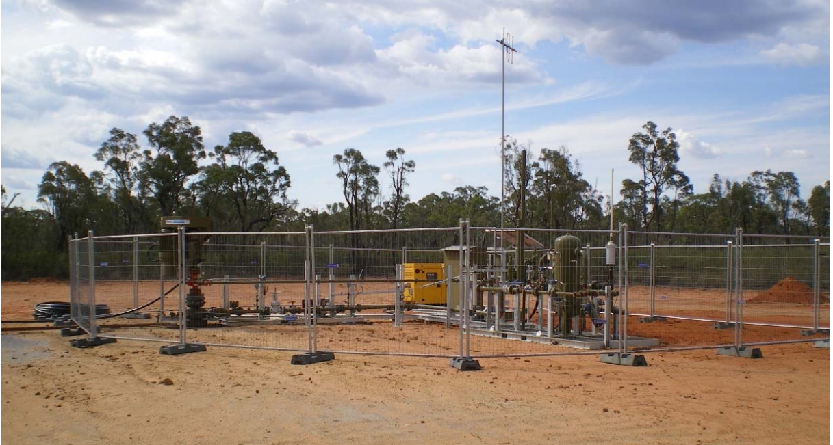
Figure 5.2-38 Typical Gas Extraction Infrastructure
