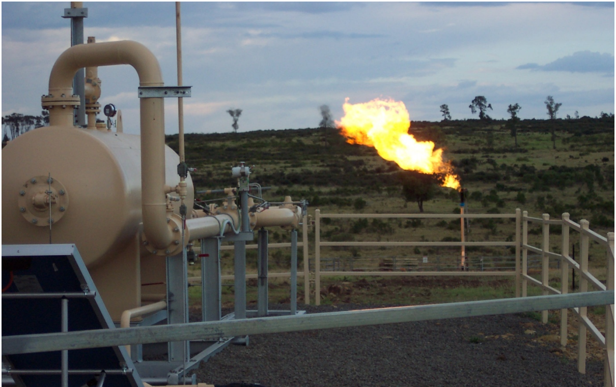
Figure 5.2-39 Typical Gas Extraction Infrastructure with Flaring
