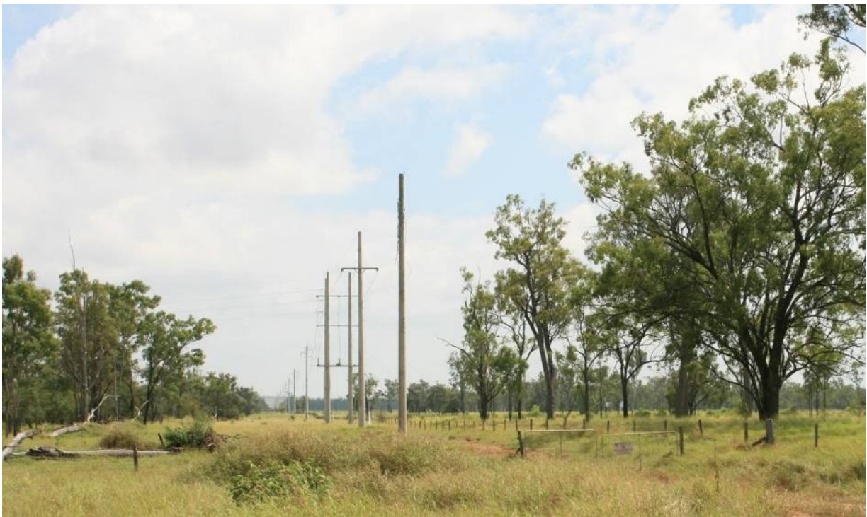
Figure 5.2-37 Typical Powerlines Associated with GRM
