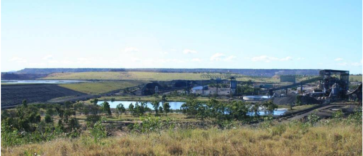
Figure 5.2-36 View of Riverside MIA and CHPP from Adjoining Reject Landform
