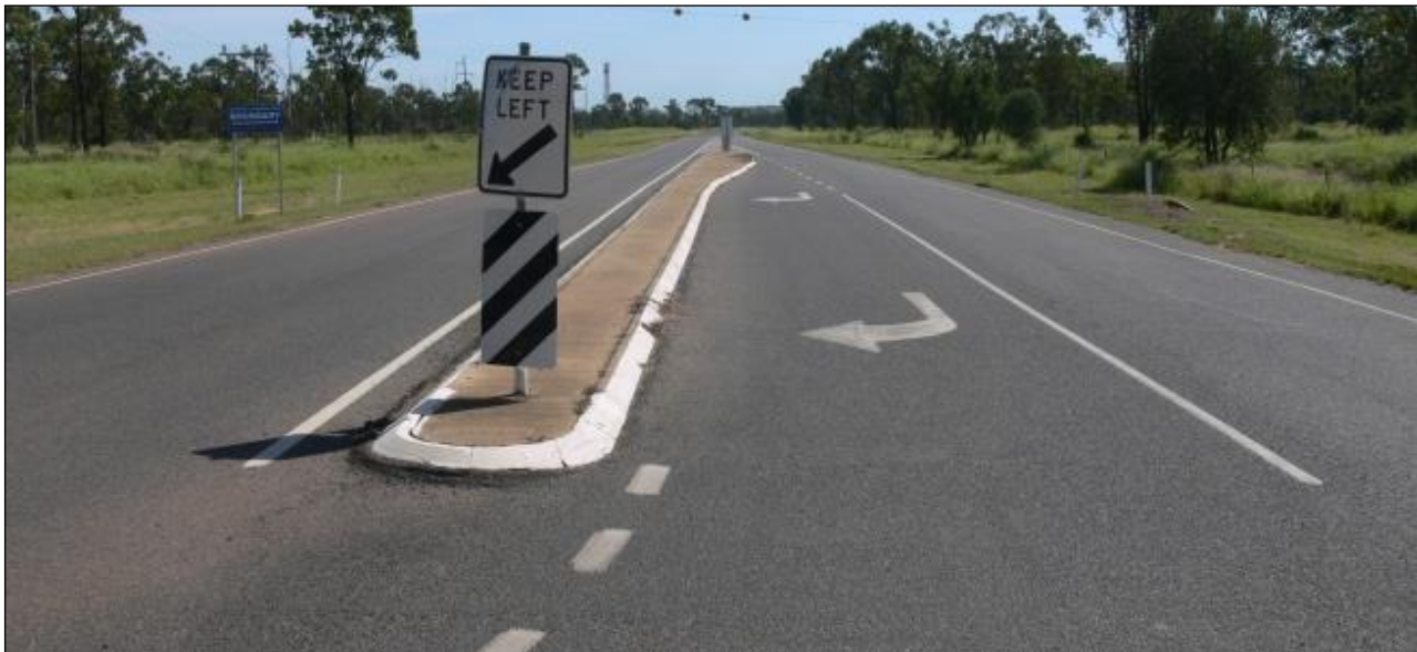
Figure 7-1 Goonyella Road/Riverside Access Road Intersection: Northern Goonyella Road Approach – Looking North
