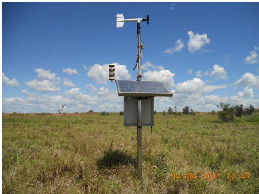
Figure 10: Northern Meteorological Station
