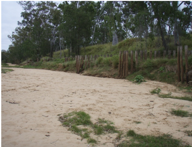
Bench maintained against toe of bank while river channel bed has deepened in response to subsidence
