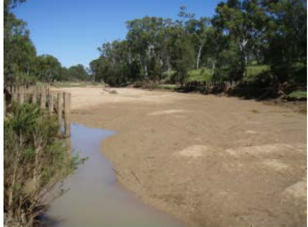
Downstream view at LW104-5 pillar zone mid 2008, note the pile fields maintaining and enhancing a bench against toe of bank
