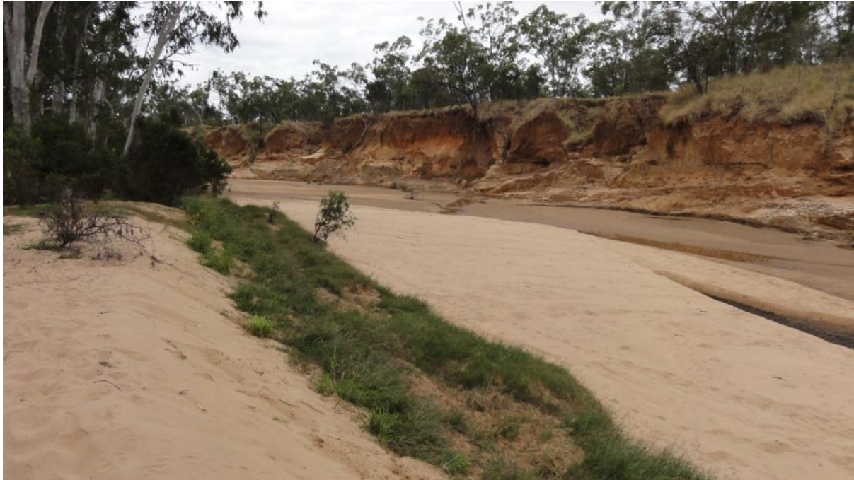
Figure 23. Existing bank instability that will be exacerbated over the main headings
