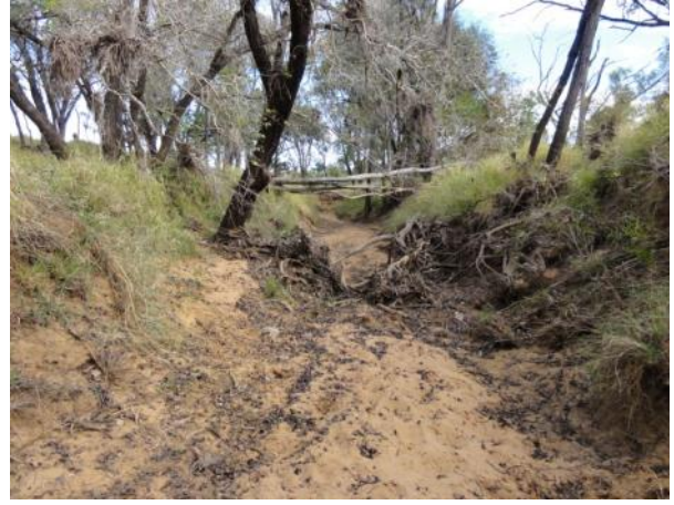
12 Mile Gully near to Mains Heading View downstream
