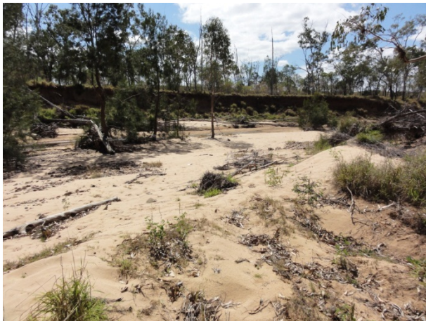
Left bank of channel subject to meander migration and flood flow re-entry erosion
