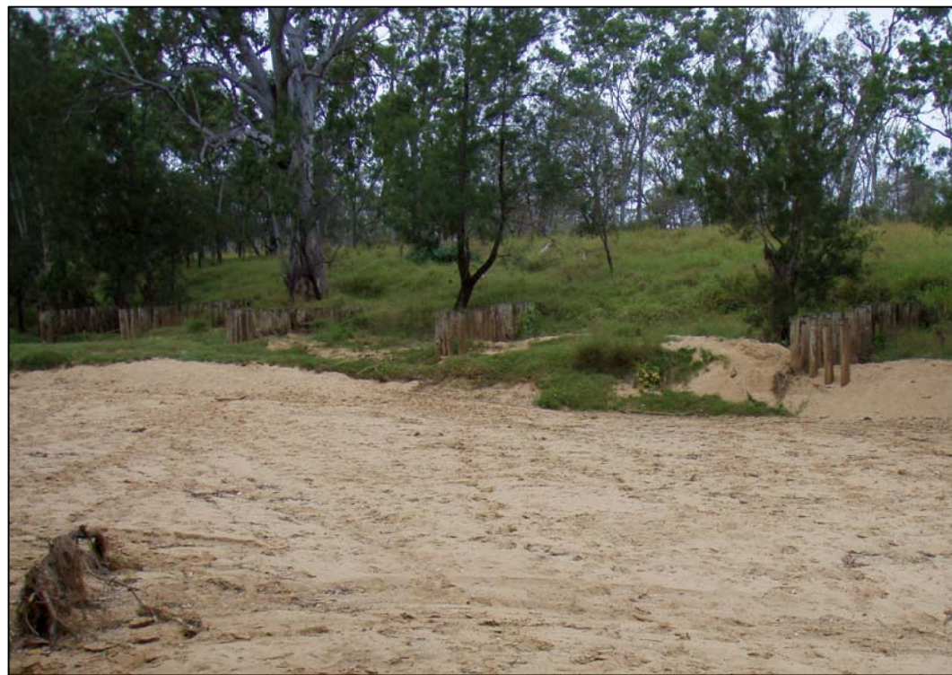
EXAMPLE – ISAAC RIVER PILE FIELDS AT BROADMEADOW MINE
