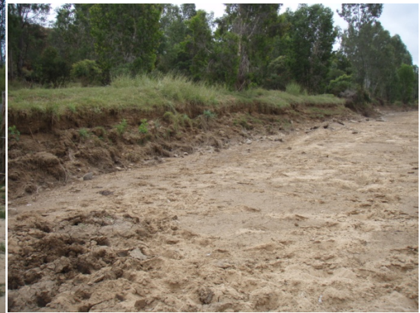
Deepening and bench erosion at LW106-7 monitoring site approximately 300m downstream of subsidence in LW105 in 2010 prior to infilling
