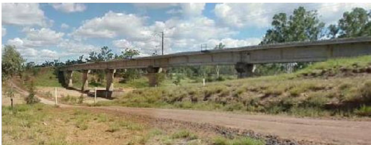
Figure 3-2 Isaac River Rail Bridge Looking Downstream
