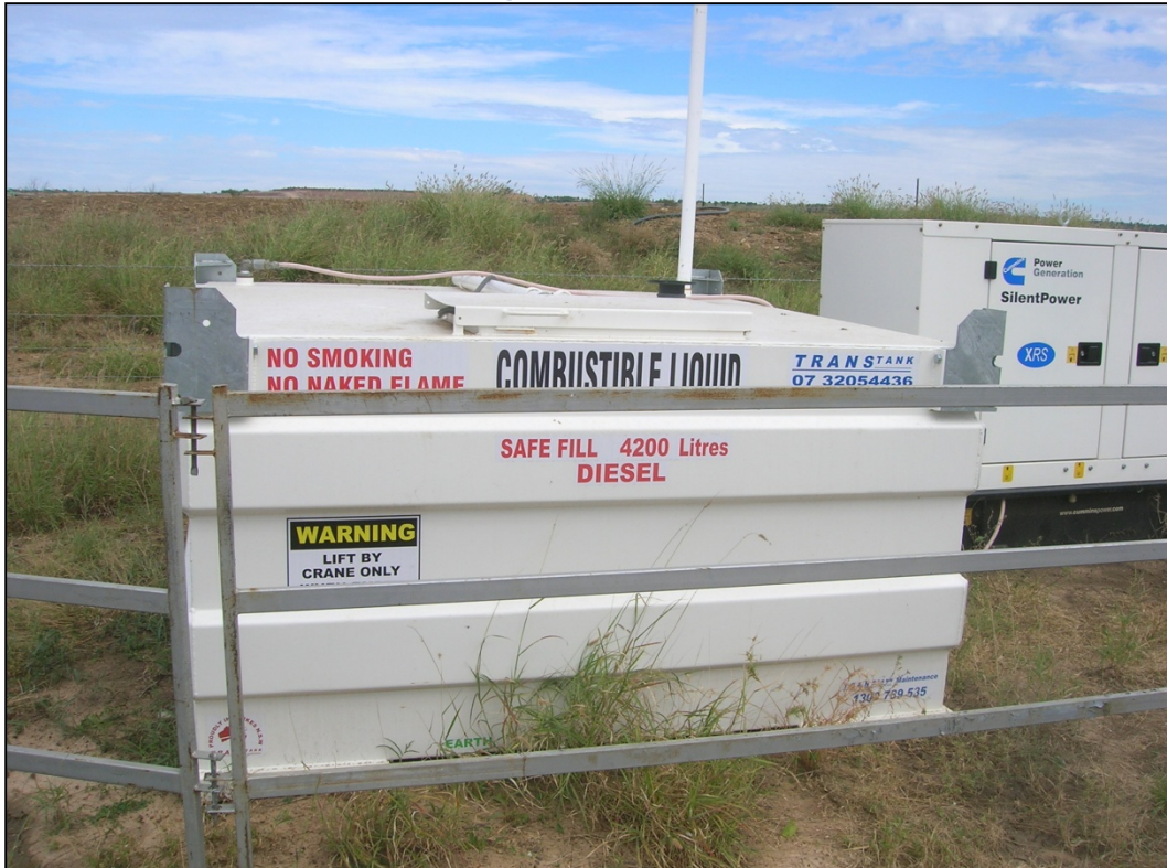
Plate B-35 Mobile Plant - Diesel Storage (2009)
