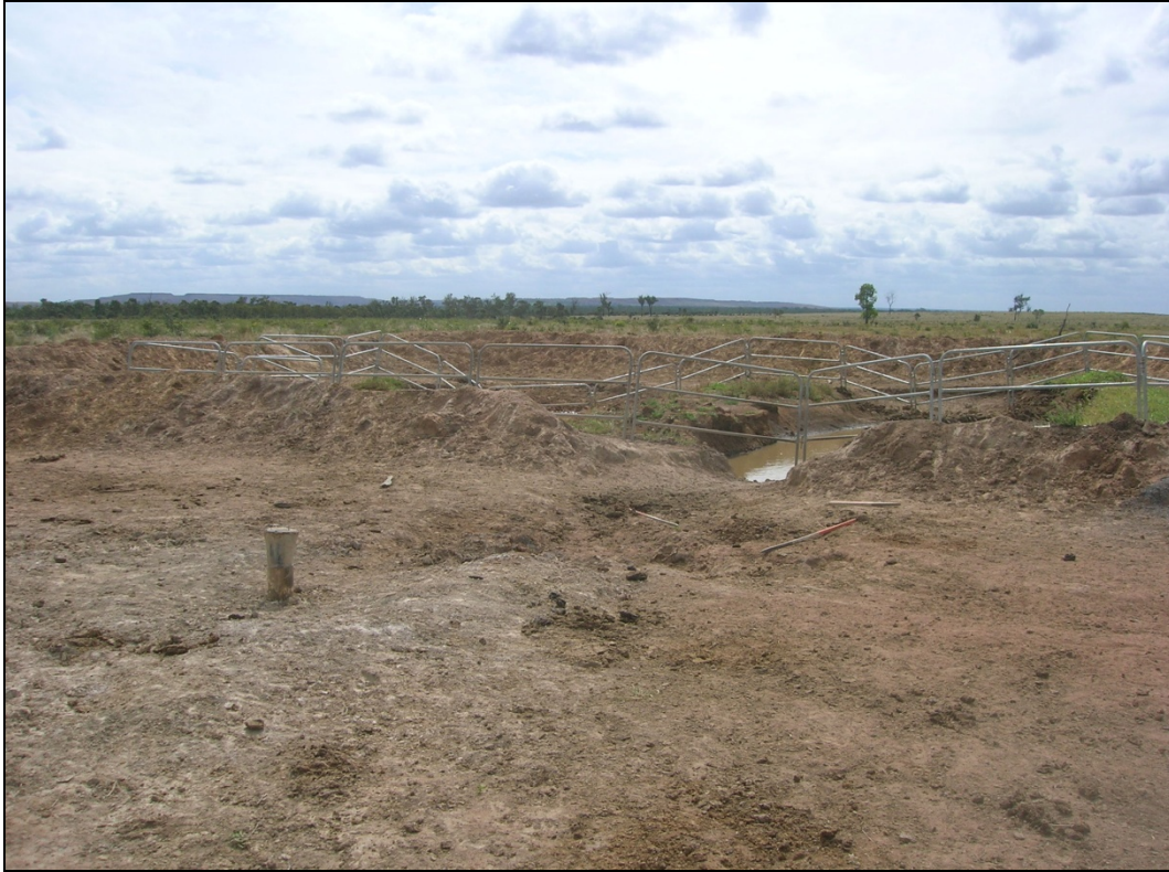
Plate B-36 Exploration Drillhole Sump - Residual Waste Water Fenced off (2009)
