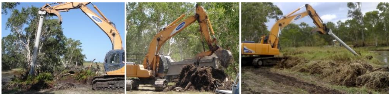
Figure 33: Removal of weed mat using an extension arm on an excavator. (Photos: A. O'Brien)
