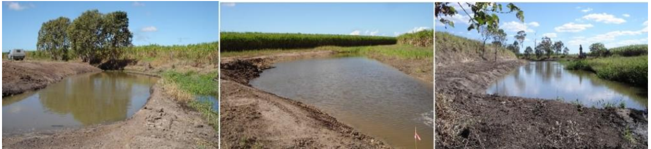
Figure 34: Three excavated detention ponds along the cane drain system. (Photos: A. O'Brien)
