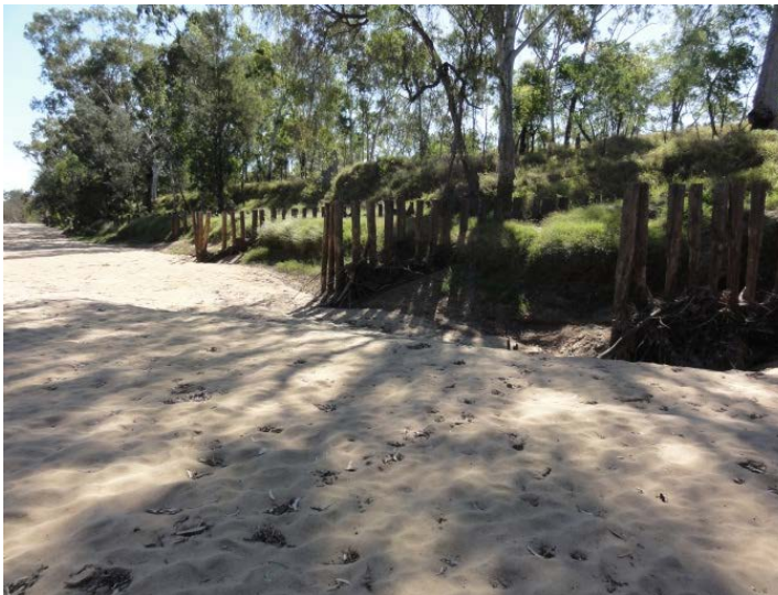
Timber pile fields at LW104-5 pillar have maintained a bench against toe of bank, mitigating the elevated bank erosion risk while both those longwalls have infilled
