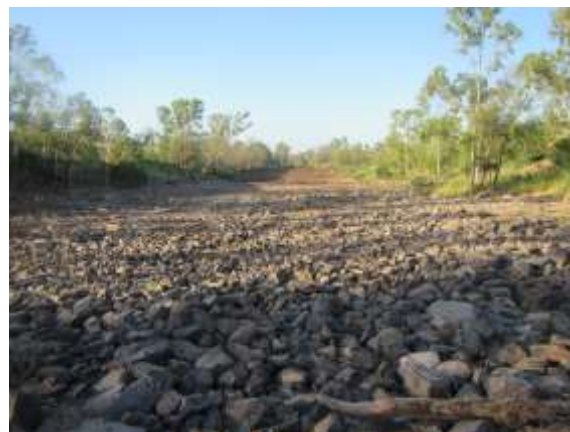
At crest of upstream drop-structuring (looking downstream at subsided LW108) following repair works
