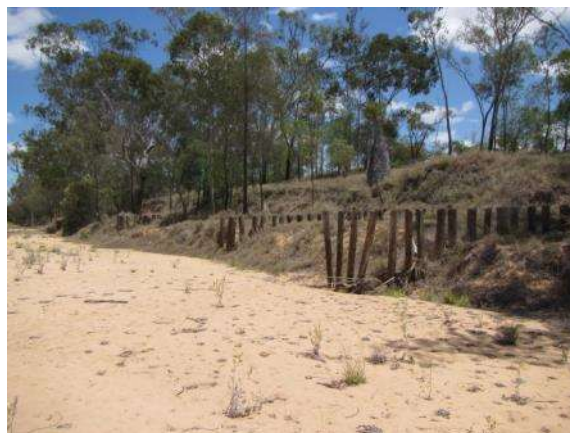
Pile fields on LW105-6 pillar zone have maintained a bench against toe of bank during the elevated erosion risk period which has now passed with infilling
