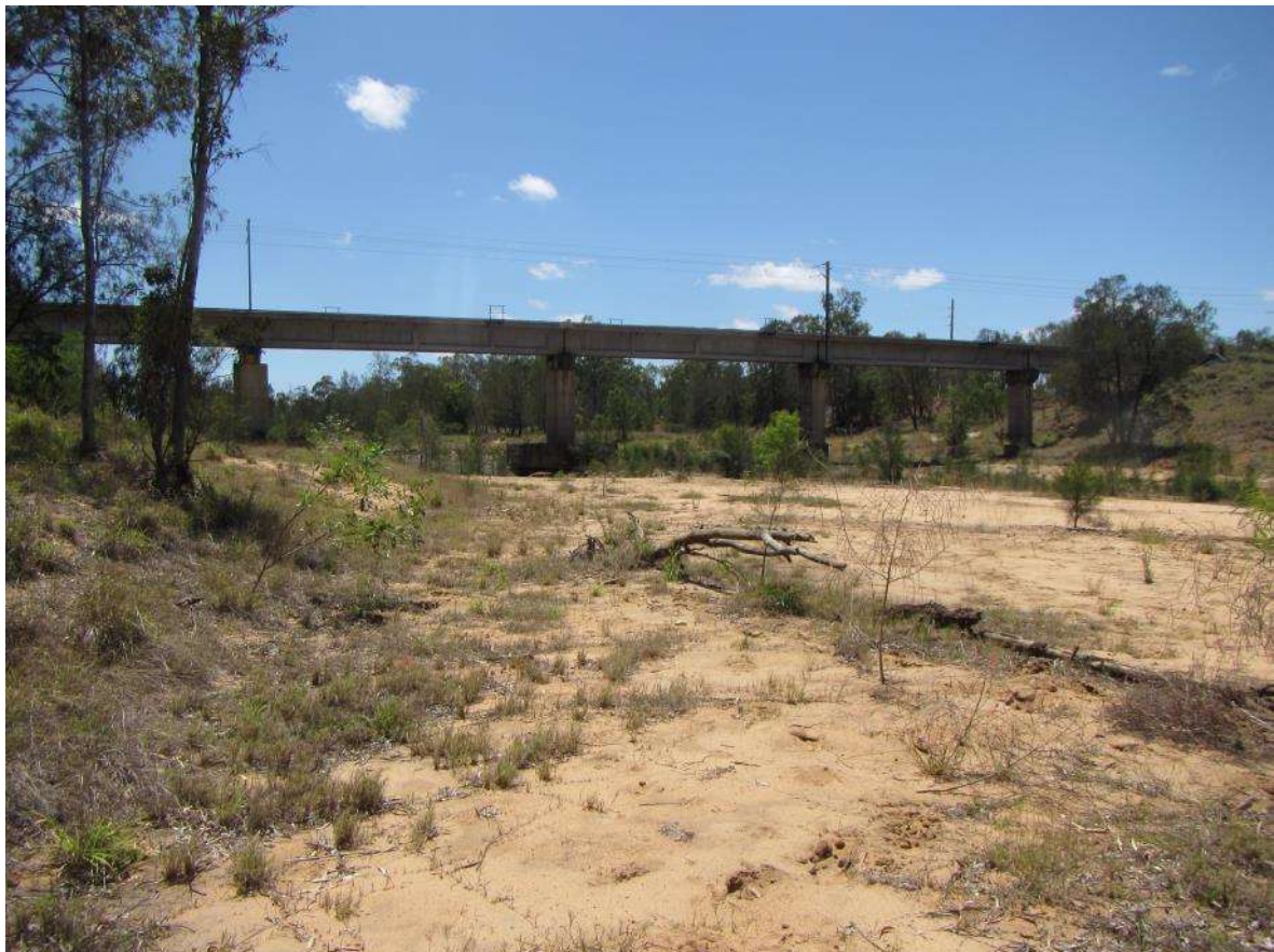
Figure 2-2: Goonyella Rail Bridge and Vehicle Crossing
