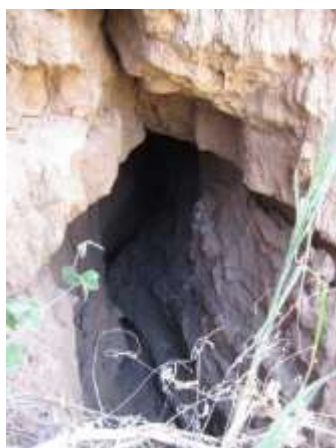
Significant worsening of tunnel erosion upstream of LW106-7 near the helipad
