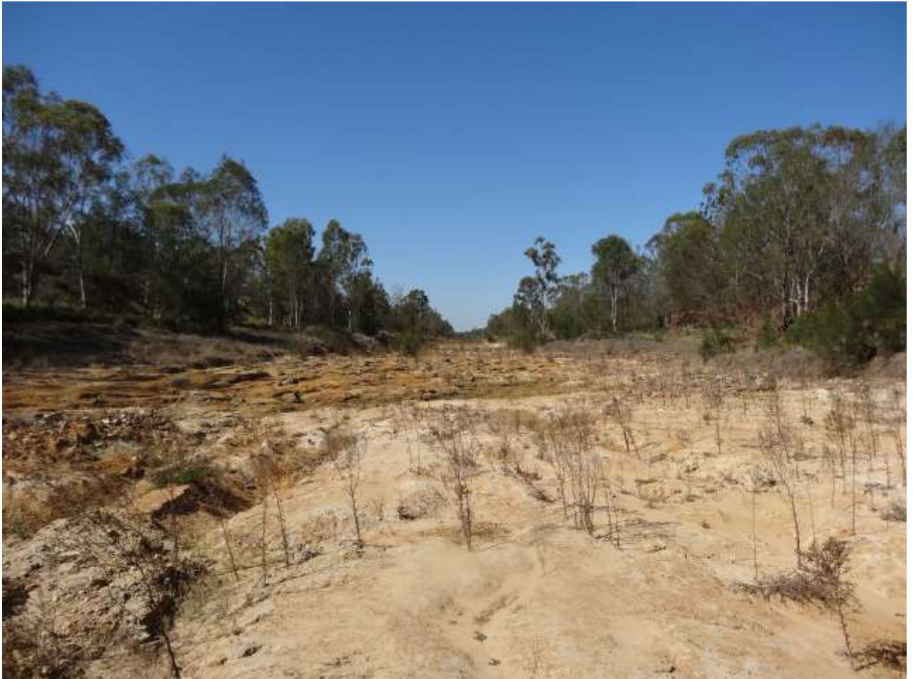
Figure 3-26: Channel bed stripped to weathered weak bedrock and clays
