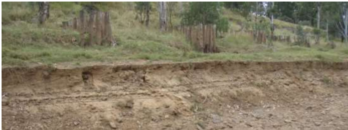
Figure 3-16: Deepening of approximately 1.5m observed over pillar LW105-06 (2010 monitoring)
