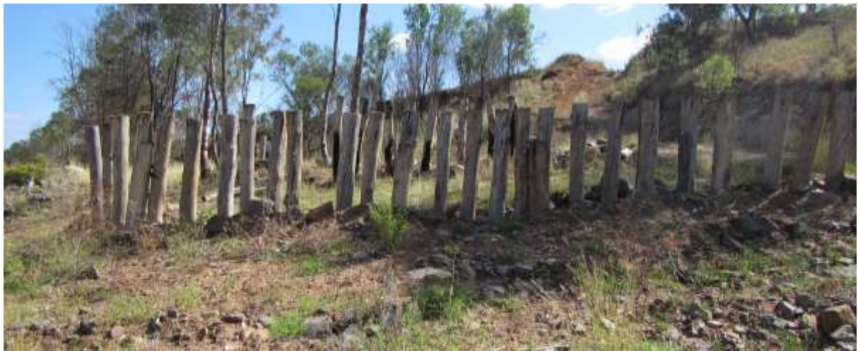
Figure 3-27: Photographs of bank erosion management pile fields implemented at BRM
