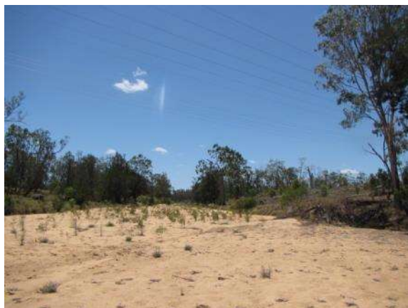
Corridor cleared for high voltage power lines
