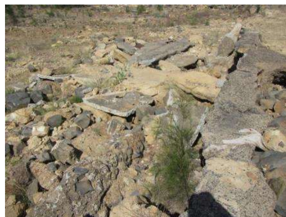
Filling of adjacent scour hole at downstream rock structure
