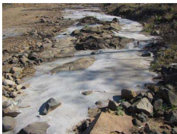
Grouting of sandstone bedrock cracking at longwall panel LW108
