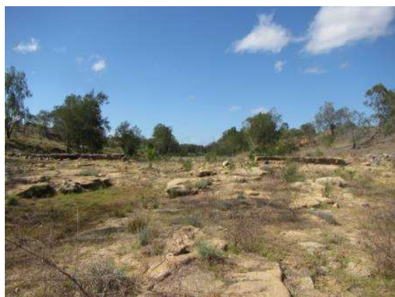
Centre of proud downstream drop structure cut-off wall removed to reduce flow concentration against banks and used to fill adjacent scour holes
