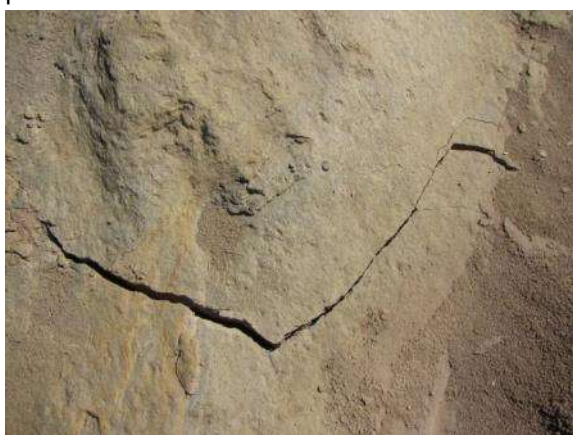
Cracking of sandstone bedrock at longwall panel LW108
