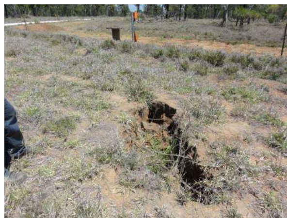
Recent crack over pillar zone between LW106 and 107 in lighter soils associated with RE11.3.2 Poplar Box association (2012)
