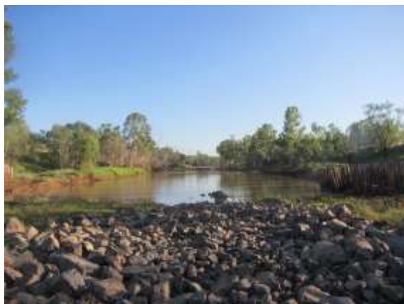
At crest of upstream drop-structuring (looking upstream) following repair works. Pool in LW107
