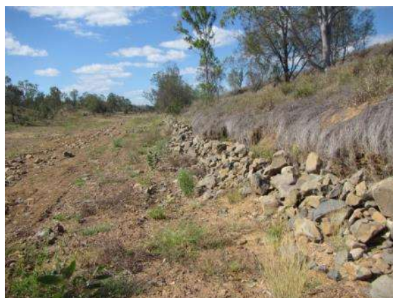
Works undertaken in channel bed to fill erosion heads and armour toe of bank with liberated rock from previous drop structure damage in subsided panel LW108
