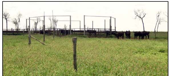
Plate 10: S View. Timber and steel cattle yards and trough.
