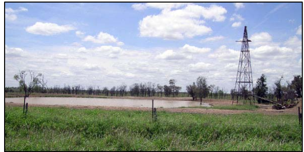
Plate 9: SE View. Damaged windmill and one of 2 nearby dams.
