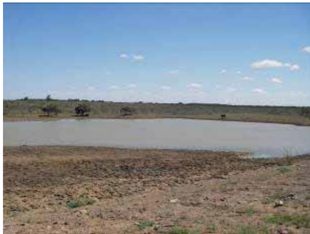
Dam looking upstream
