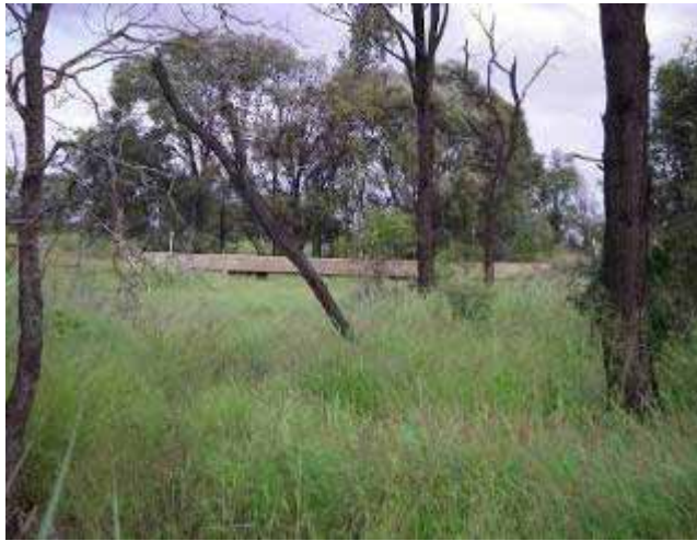
Culvert crossing Peak Downs Highway
