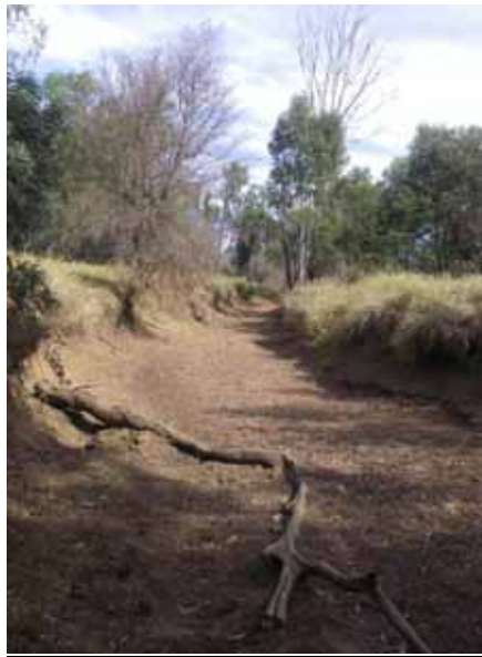
Looking upstream from road crossing
