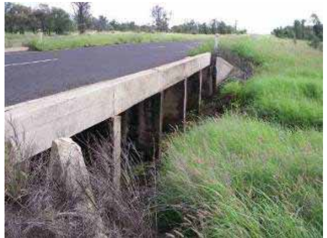
Five box culverts
