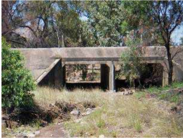
Horse Creek crossing culverts, looking downstream
