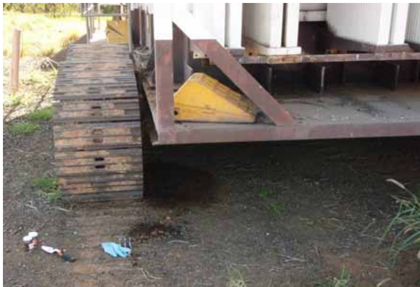
Plate 30 Oily stain under Transformer TSS01 – Peak Downs Mine
