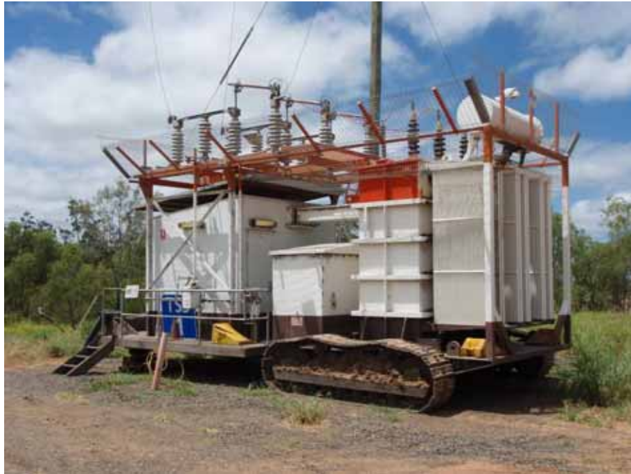
Plate 27 Mobile Dragline Transformer - Peak Downs Mine
