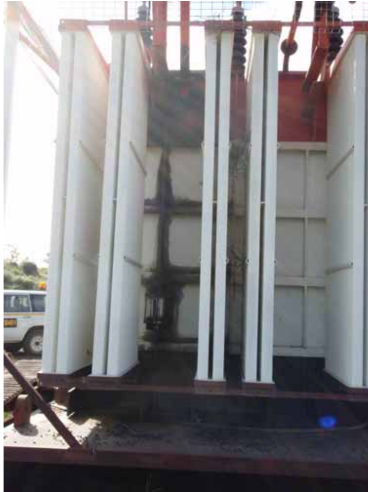
Plate 29 Oily Staining on Windings case on Transformer – Peak Downs Mine
