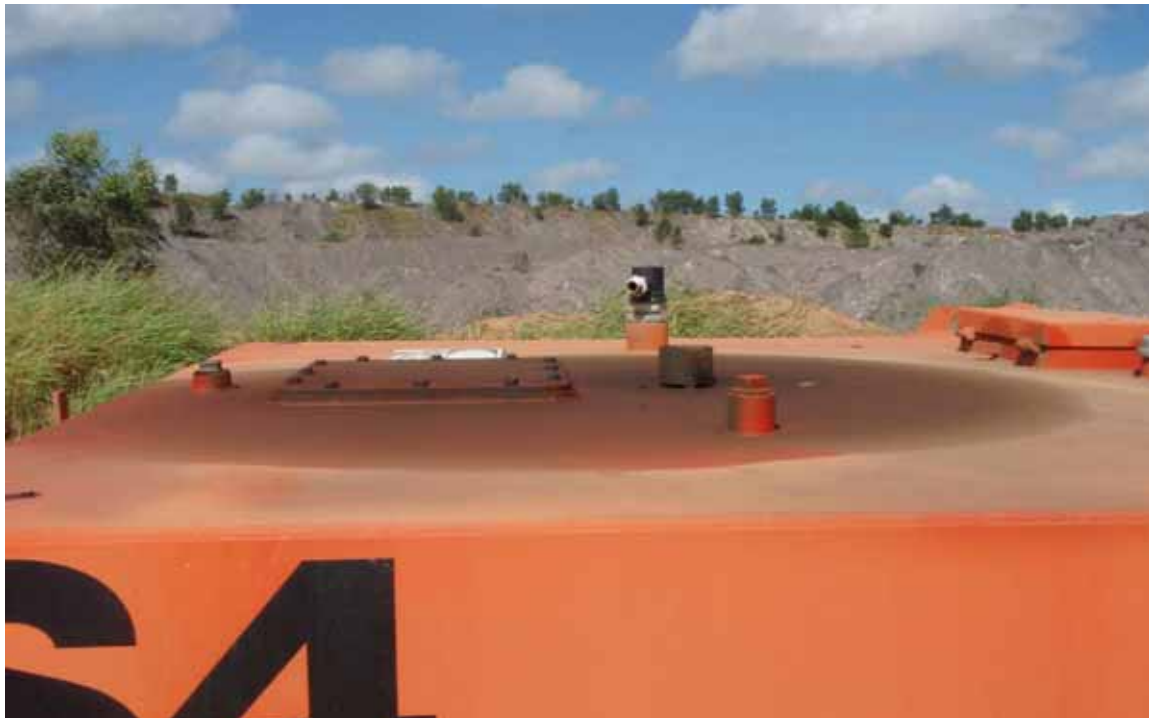
Plate 32 Staining on tank fill point – Peak Downs Mine
