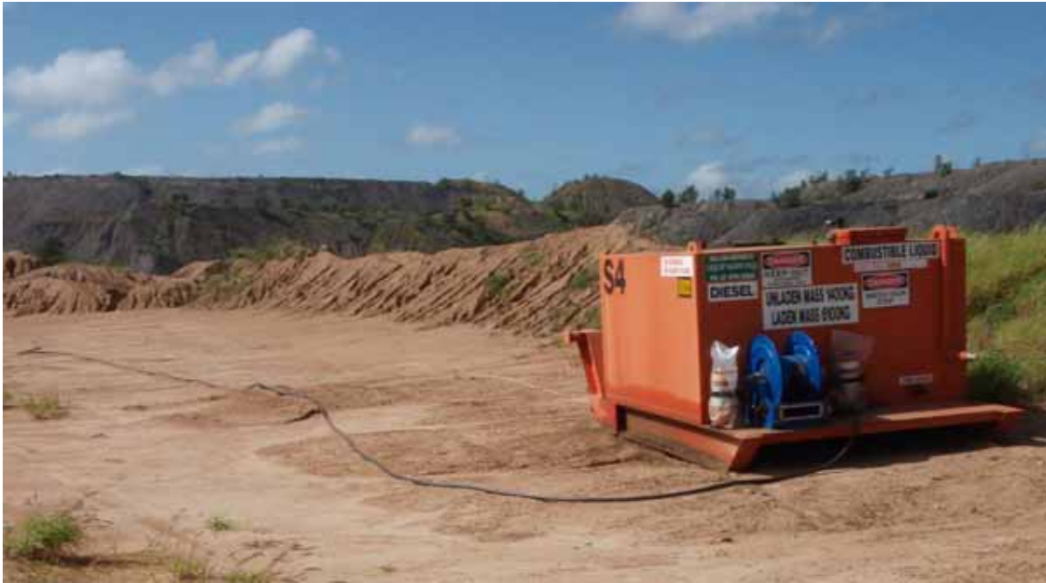
Plate 31 Diesel Fuel tank at 11North Pit –Peak Downs Mine
