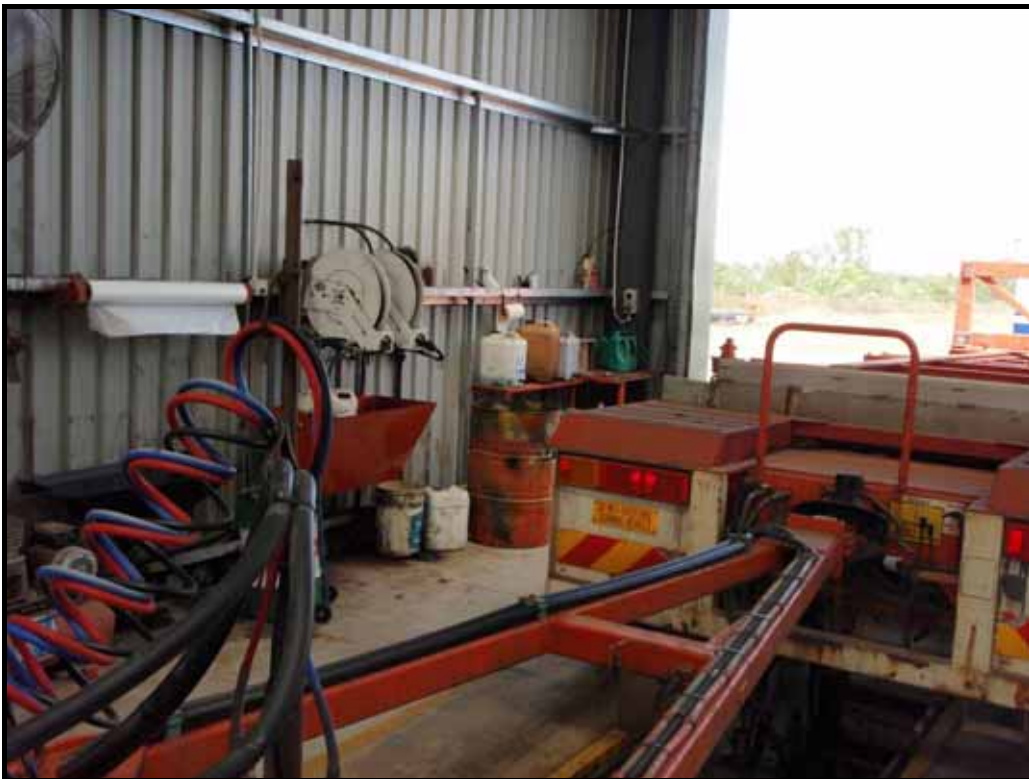
Plate 16 Workbench and lubrication filling - Kalari Yard
