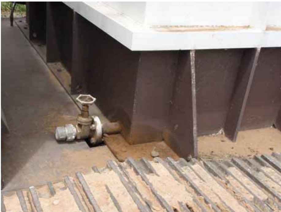
Plate 28 Oily Staining on Spigot on Transformer – Peak Downs Mine
