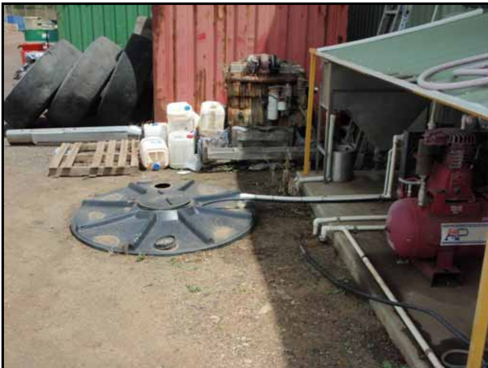
Plate 4 In-ground Waste Oily Water/sediment tank - Kalari Yard
