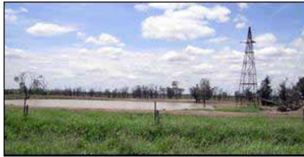
Figure 3.10.4 South-East View. Damaged Windmill and a Nearby Dam.
