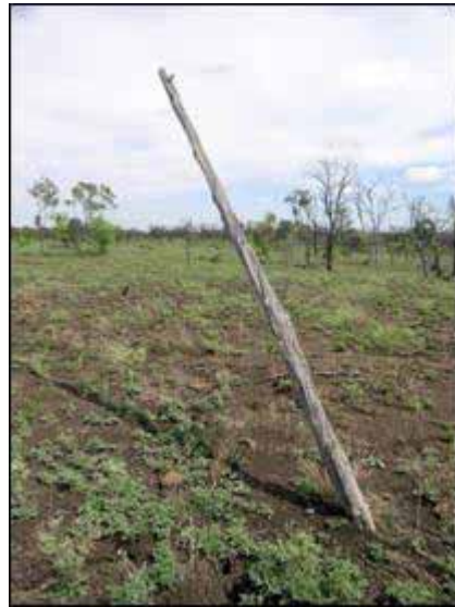
Figure 3.10.2 North View. Telegraph Post
