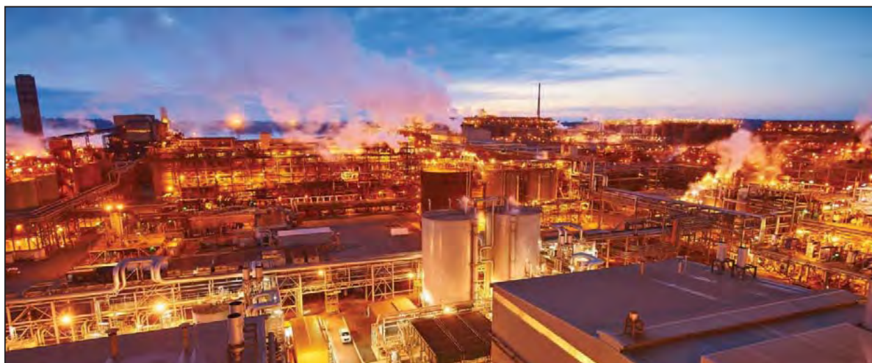
Figure 8-1: Worsley Alumina Refinery
