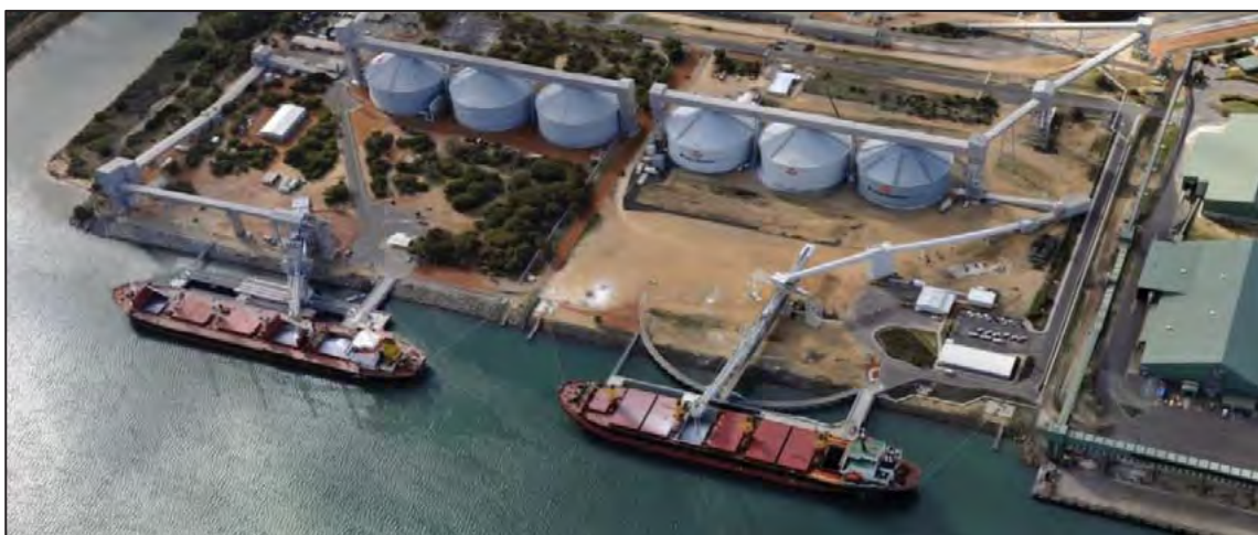
Figure 9-2: Worsley Alumina port facility (right side)
