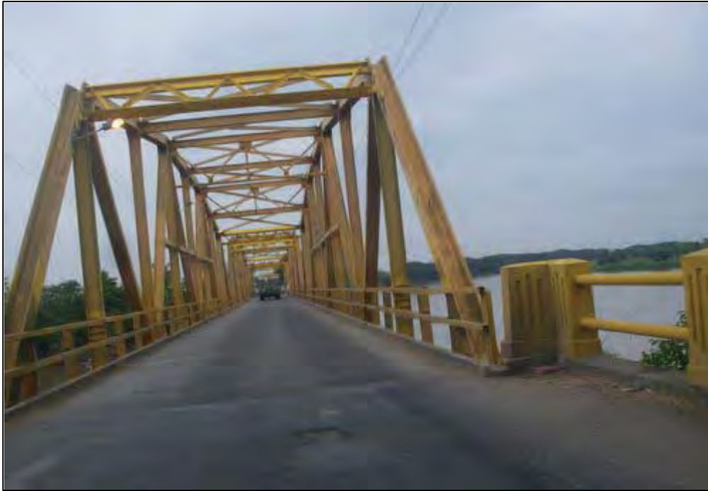
Figure 9-2: Existing bridge over the St George River
