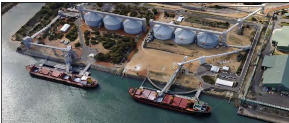
Figure 9-2: Worsley Alumina port facility (right side)
