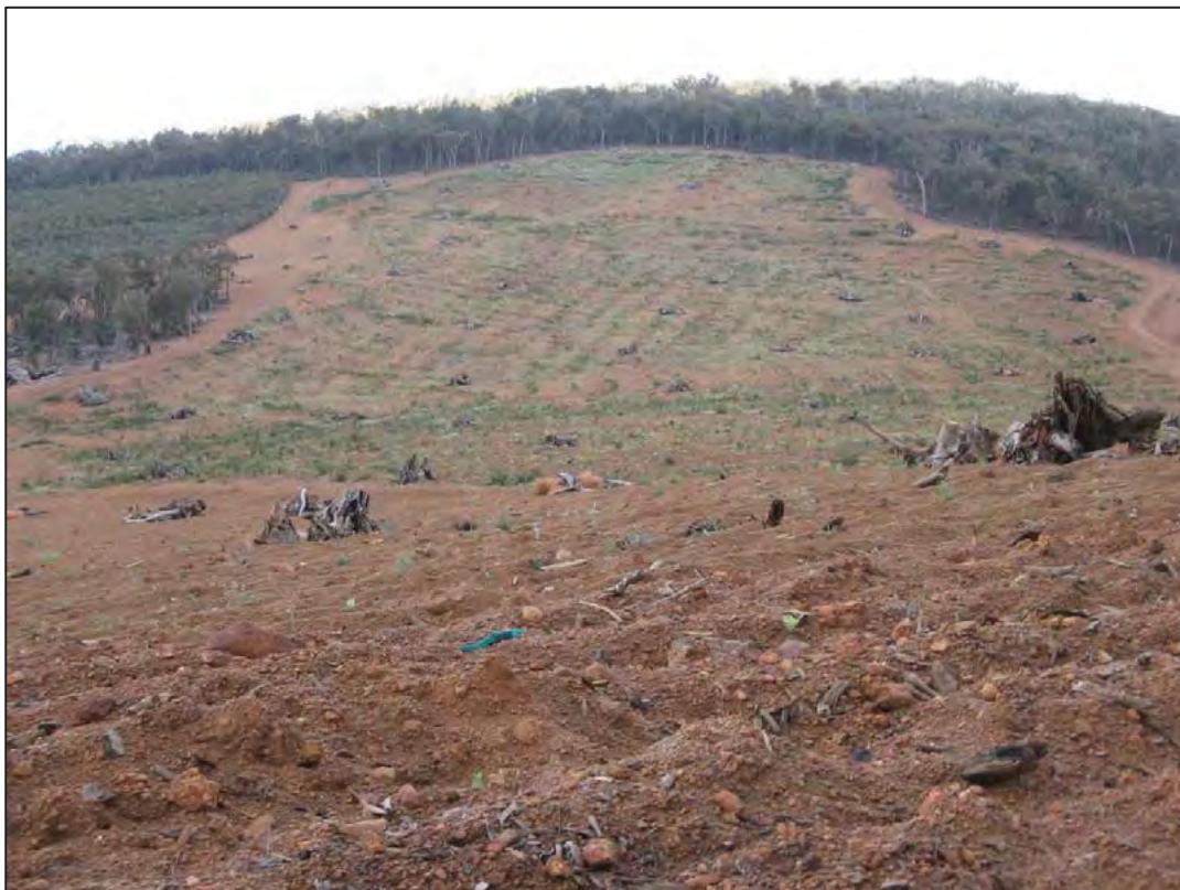
Figure 7-6: Backfilled mined out area with topsoil and reclamation area in background – Saddleback area
