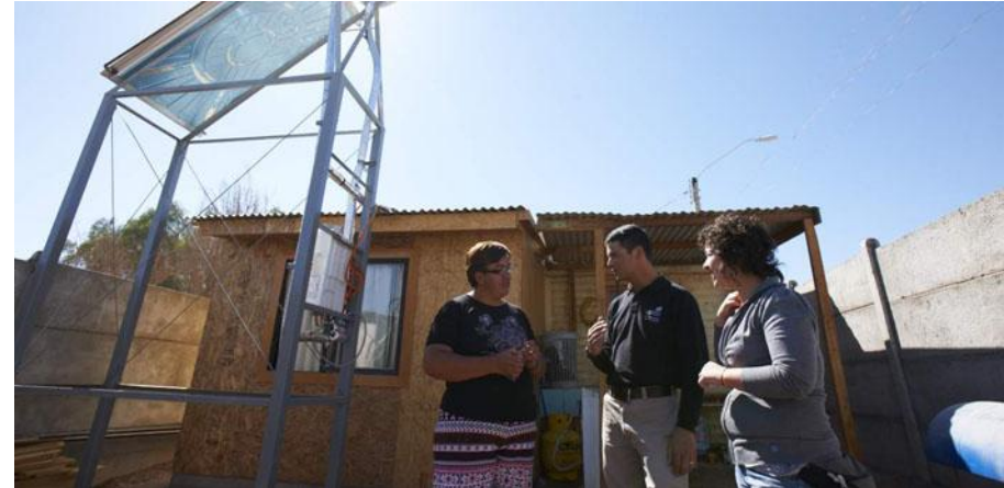
Installing solar panels in local homes, Spence Base Metals, Chile
