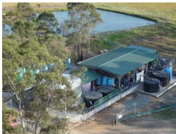
The water filtration plant at our Illawarra Coal Appin West site.
