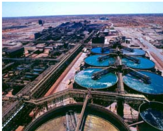
The Concentrator/Hydromet Plant at Olympic Dam where significant water savings have been identified.
