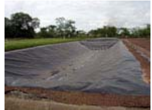
A sanitary landfill facility has been constructed.
