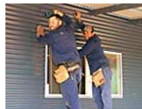
Another job under way for apprentices from Meta Maya Building Services, which provides residential property services.
