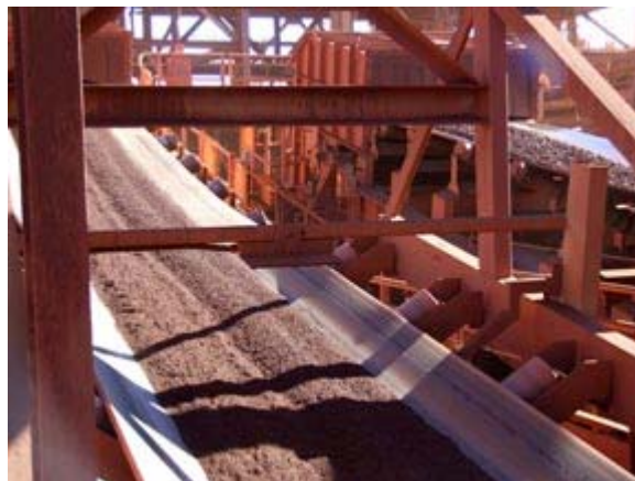
Low-frequency microwave moisture analyser in use.
