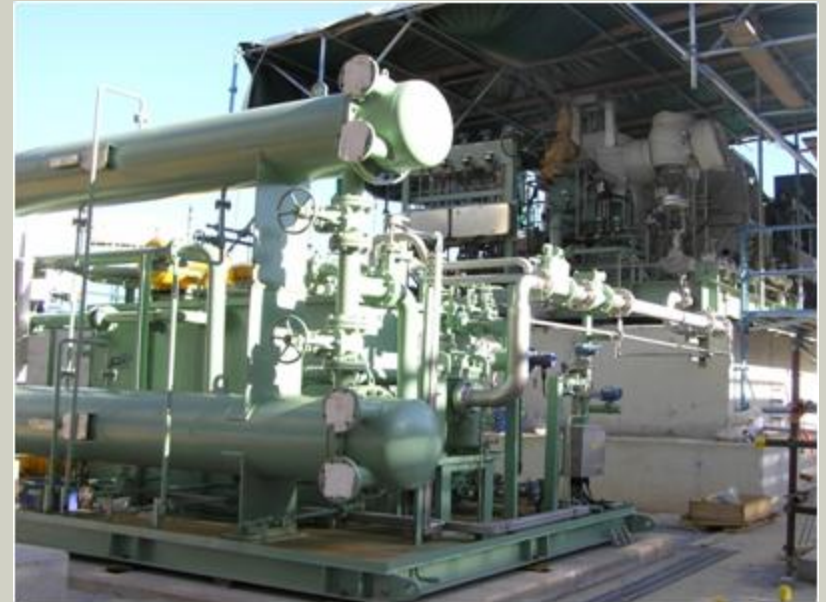
Power plant steam blowing main header
