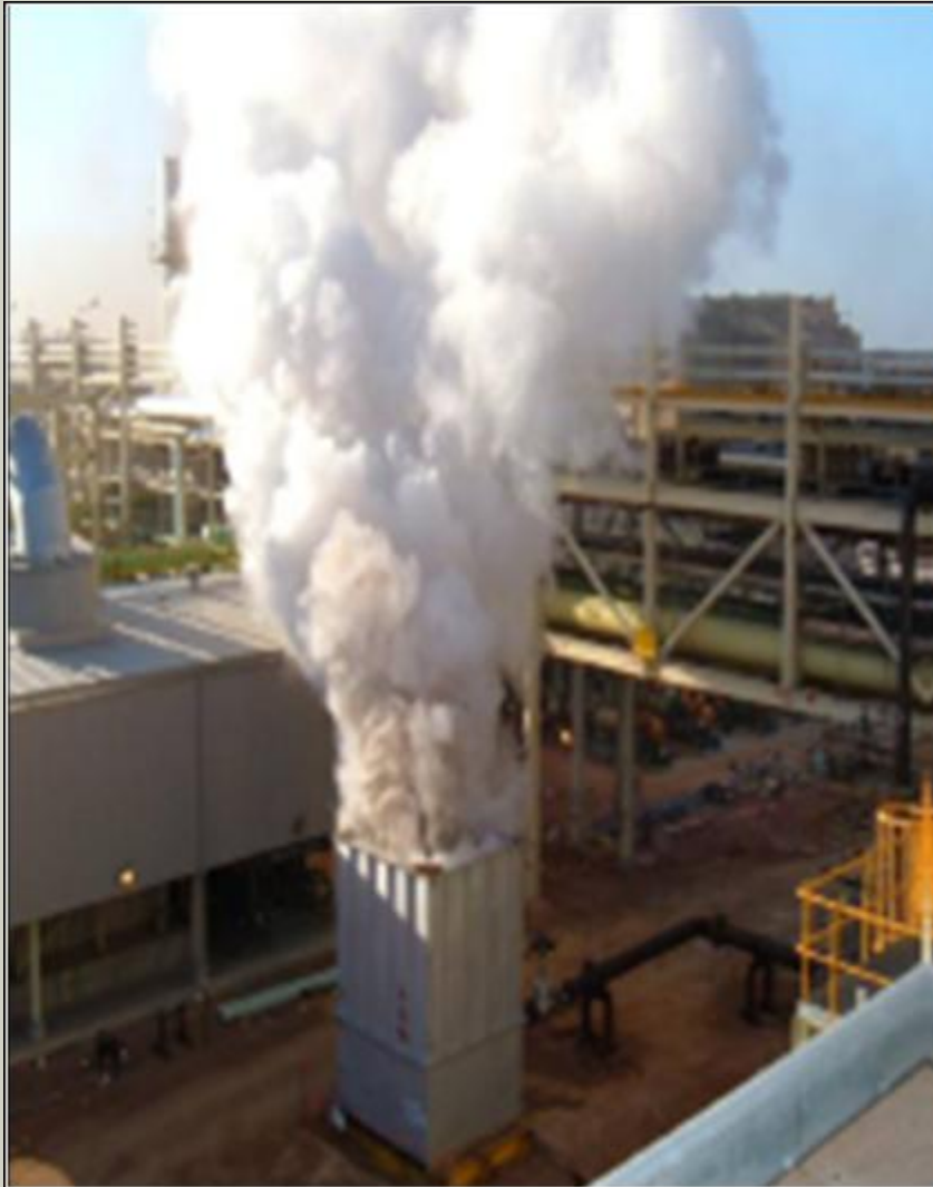
Power plant steam blowing main header
