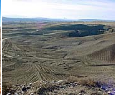
Reclamation of Cottonwood Pit prior to topsoil
