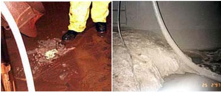
Typical accumulation on the bottom of tanks
