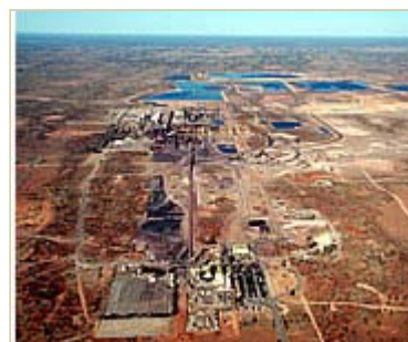
Aerial view of Olympic Dam operation with the mine in the foreground and the processing plant and tailings storage facility in the background
