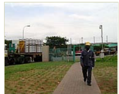
Pedestrian walkway constructed as a safety measure
