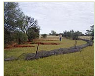
Intervention to address erosion, April 2006
