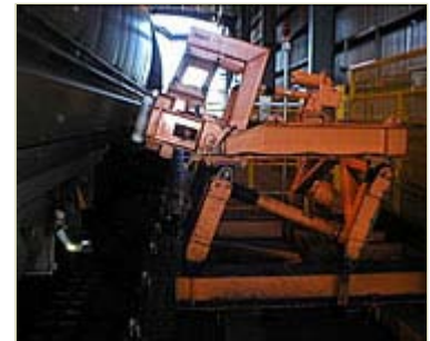
A wagon vibrator in action at the Hay Point coal terminal
