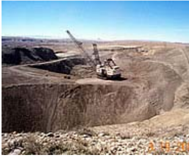
Start of reclamation of Cottonwood Pit at San Juan Mine
