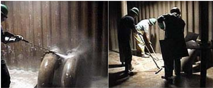
Typical accumulation on the bottom of tanks.
