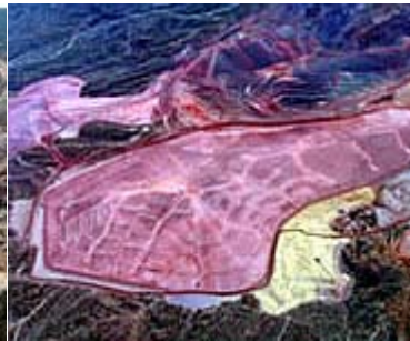
Reclamation under way in 2005
