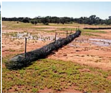
Intervention to address washaways, April 2006
