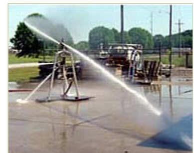
Using high-pressure hydraulic jets perform significantly reduces potential safety issues
