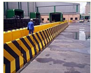
Protected walkway constructed as a safety measure
