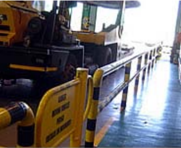
Barriers in mobile equipment workshop for safer pedestrian movement
