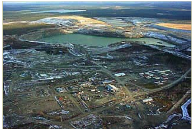
Selbaie after demolition, November 2004
