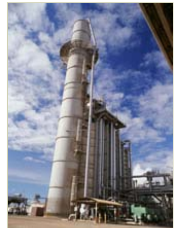
Worsley's gas-fired cogeneration plant
