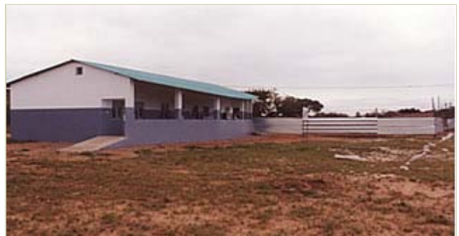
Maternity facility at the Beluluane Clinic
