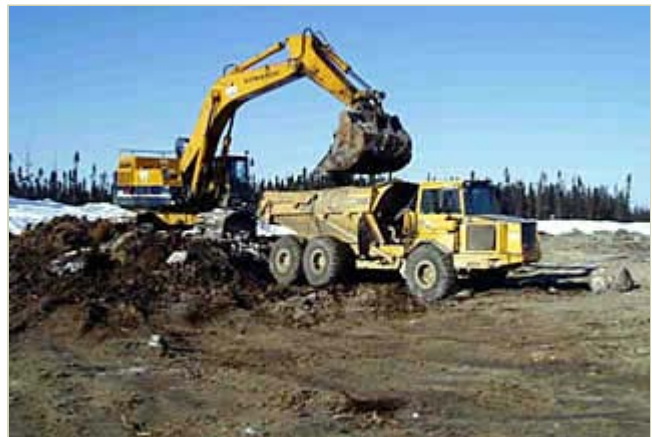
West Sector – removal of frozen contaminated peat for disposal and treatment in open pit – February 2005
