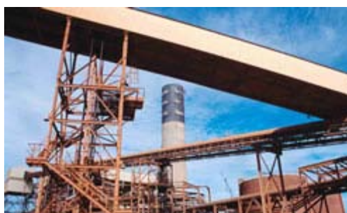
Worsley Alumina Refinery
