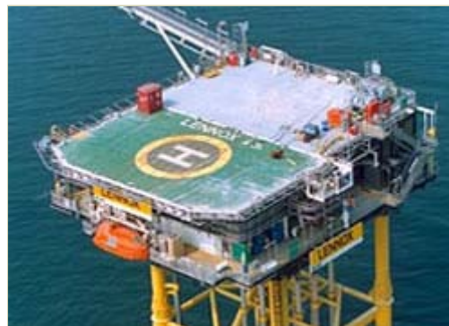
Liverpool Bay Lennox satellite platform at Liverpool Bay, UK
