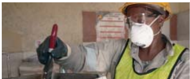
► Maduka Construction employee working on stonedust barrier
