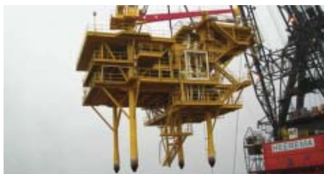
► The Kairi 1 offshore platform constructed by local company Damus Ltd
