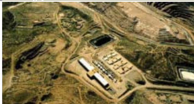
► Aerial view of the San Manuel mine site
