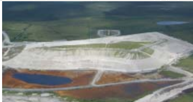
► Waste rock pile at Selbaie Mine with acid collection pond in the foreground. The area of release from ditches is in the top right corner.
