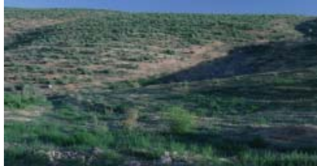
► Reclaimed southern slope of the McDermott Dump located at the east end of La Plata Mine. The dump was reclaimed in 2001 using fluvial geomorphic principles to design the size, shape and features of the watershed.
