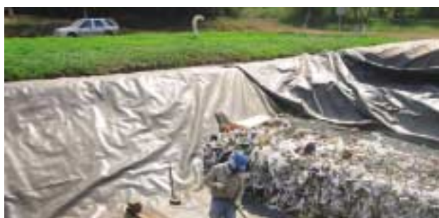
► Solid waste disposal site at Montelíbano
