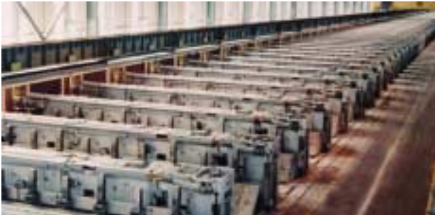
► Potroom at Hillside smelter
