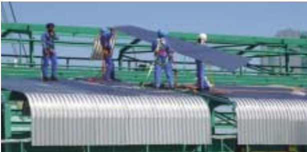
► Construction of potroom, Mozal 2 expansion project
