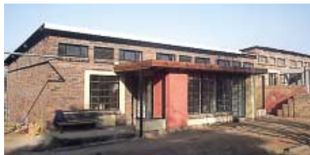
► Metalloys hostel under conversion to the Kotulong community support centre
