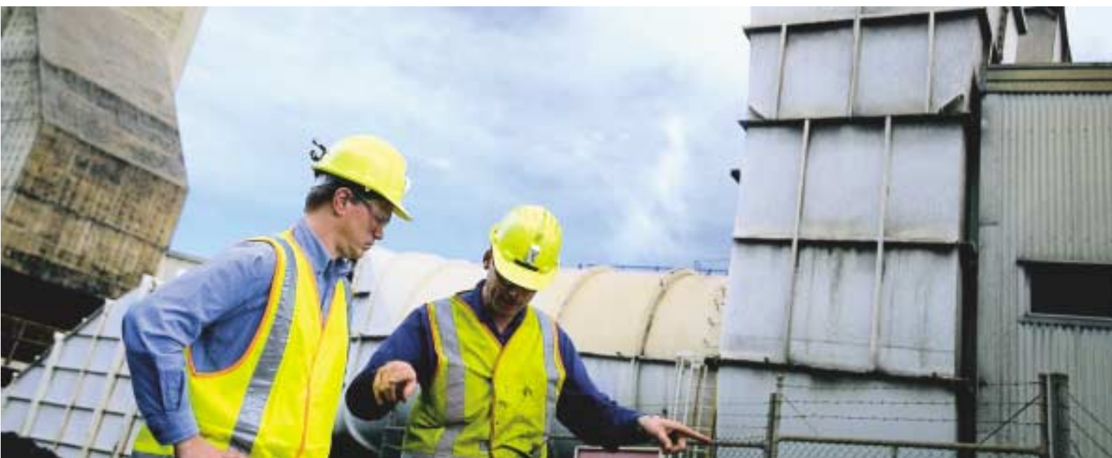
Richard Danell, Project Leader, and Roger Bowman, Coal Preparation Manager, plan the linkage from West Cliff Colliery's mine air ventilation exhaust duct to the new methane utilisation plant
