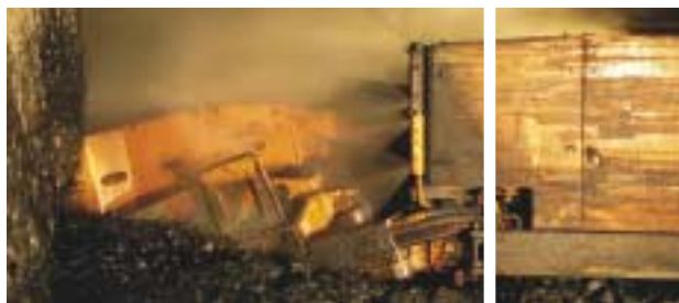
Dust suppression sprays on continuous miner, Douglas Colliery, South Africa
