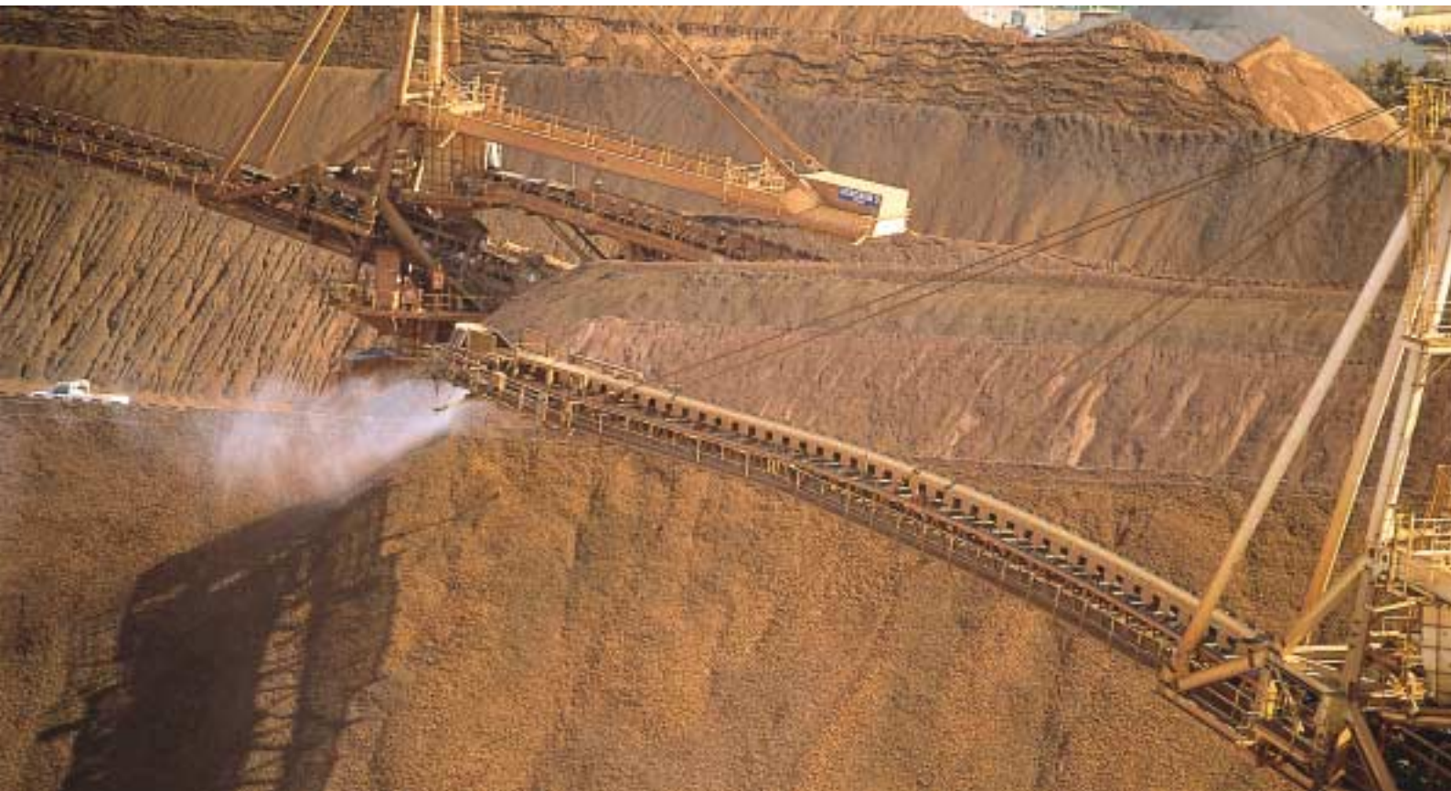
Dust suppression spray in operation at Port Hedland iron ore stockpiles
