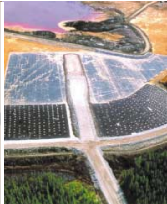
Geomembrane liner under construction, Poirier
