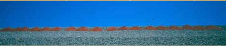
Left: Topsoil prepared for spreading on the wall of the Kambalda tailings storage facility.
