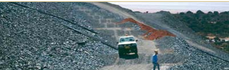
Barry Clouett, Metallurgy Manager – Kambalda Nickel Operations, inspects innovative profiling of the tailings storage facility. The new work aims to encourage rehabilitation on the slopes and limit erosion.
